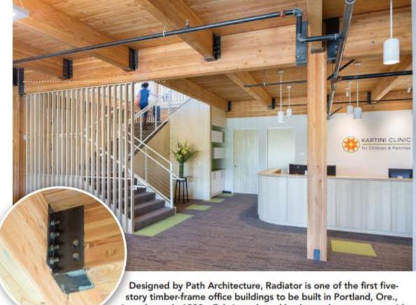
since the early 1900s. Fabricated steel bucket-style connectors with bolts were utilized for glulam beam-to-beam connections.
