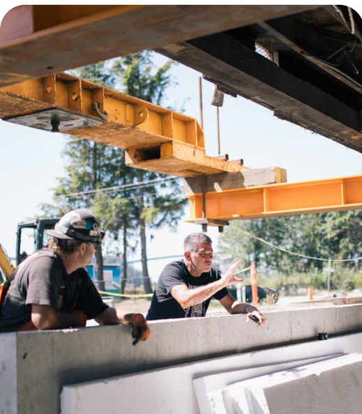
Nickel Bros. team planning to lower the LYSH onto its new foundation
