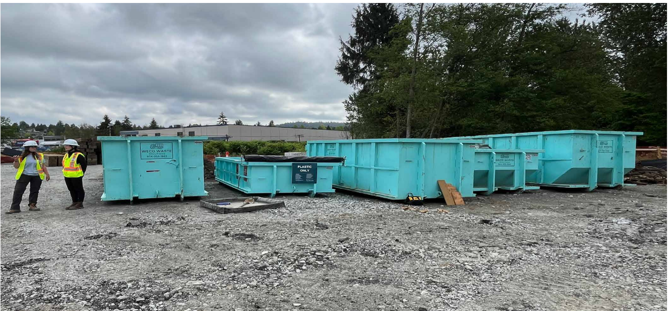
Figure 30: Plastics bin positioned on a construction site
