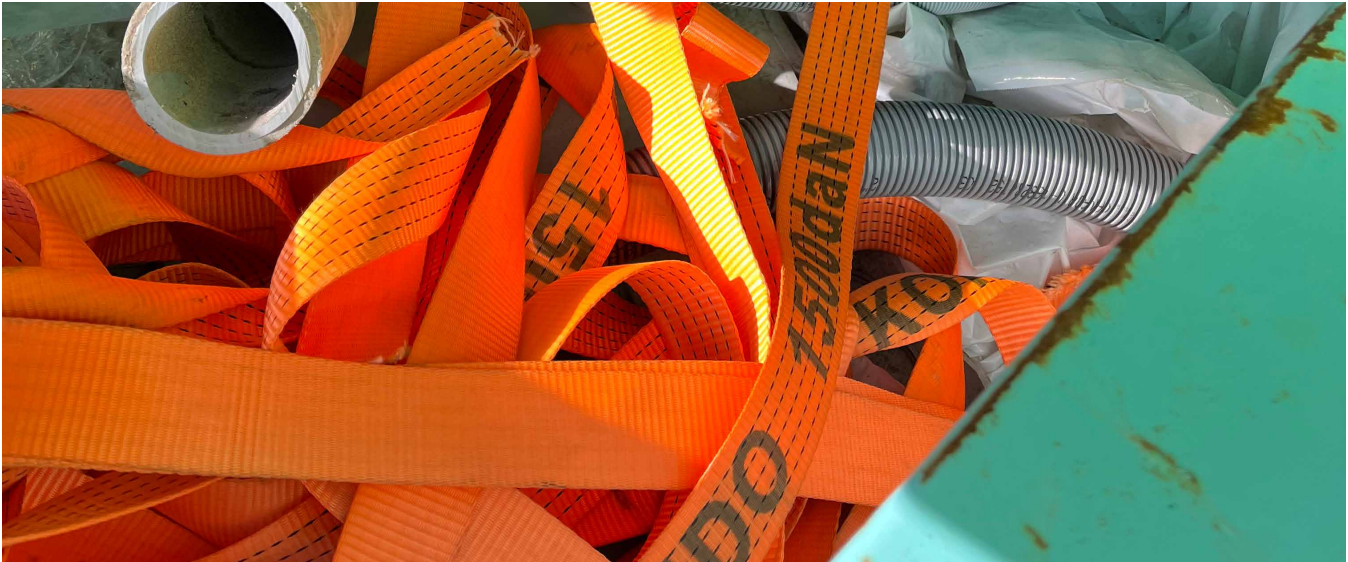
Figure 15: Plastic inside a CPI bin on a construction site
