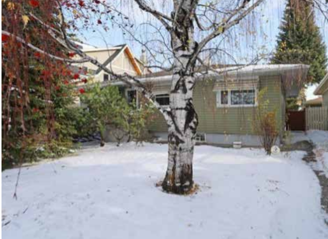
Figure 16: Calgary home pre demolition
