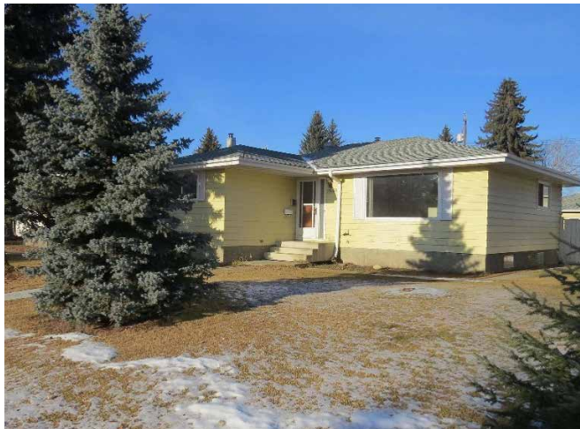
Figure 17: Edmonton home pre demolition
