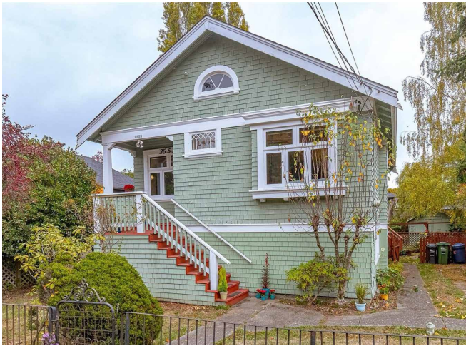
Figure 14: Victorian home pre deconstruction
