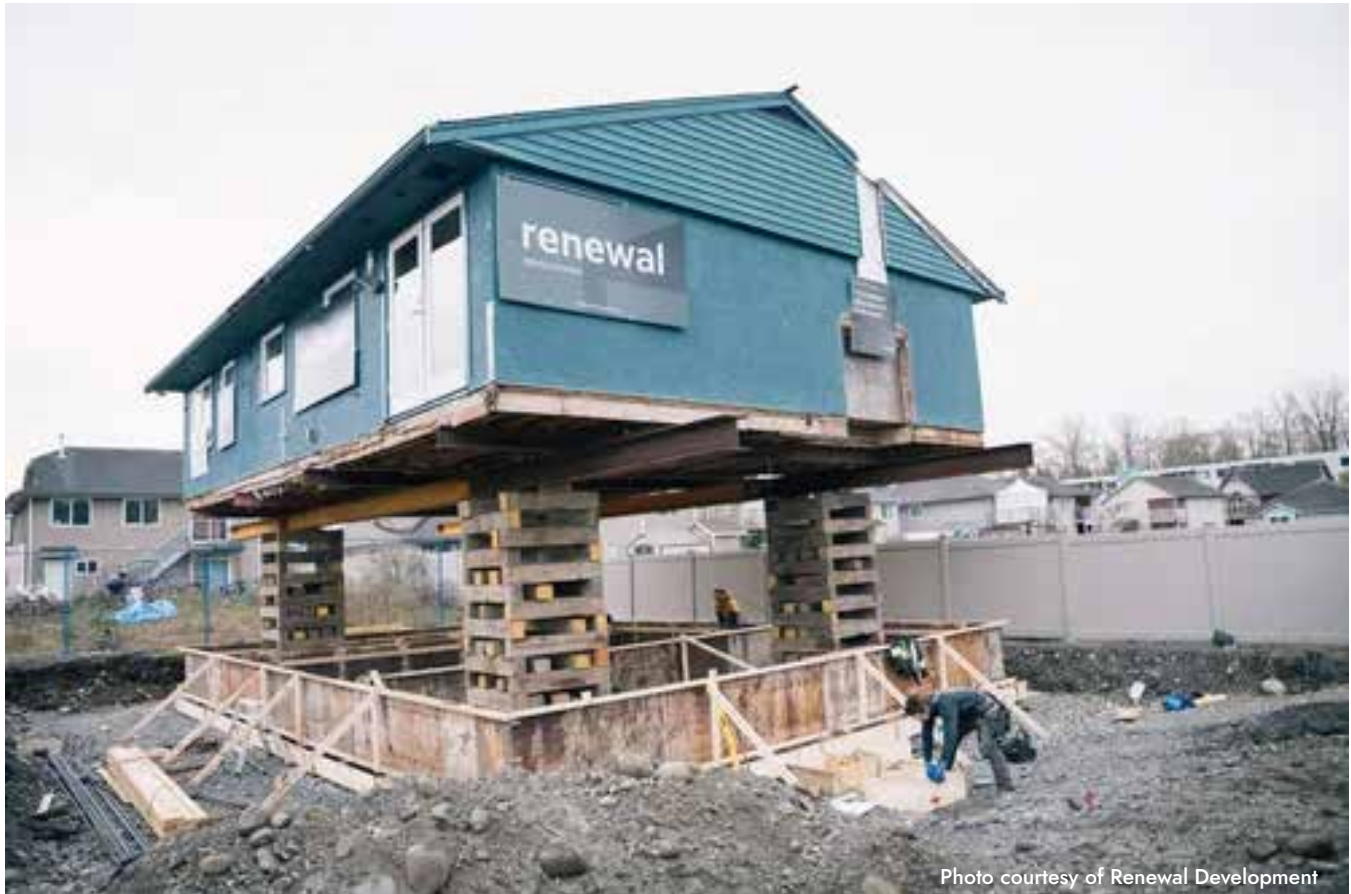
Figure 7: The Colwood home being prepared for relocation
