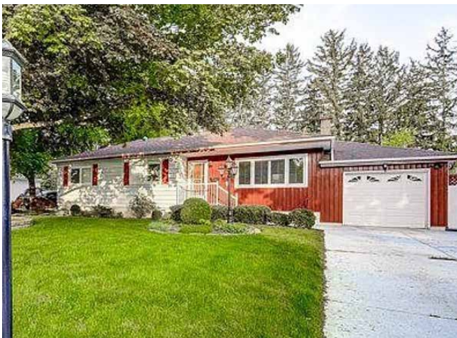
Figure 18: Hamilton home pre demolition
