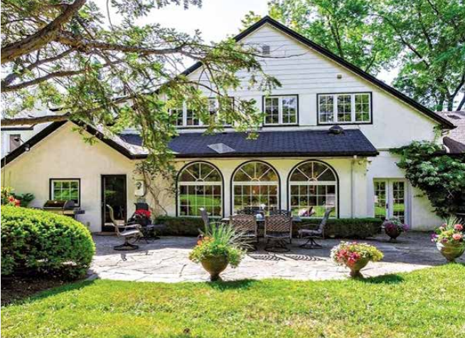
Figure 19: Toronto home pre demolition
