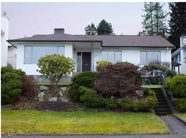
Figure 15: Vancouver home pre demolition
