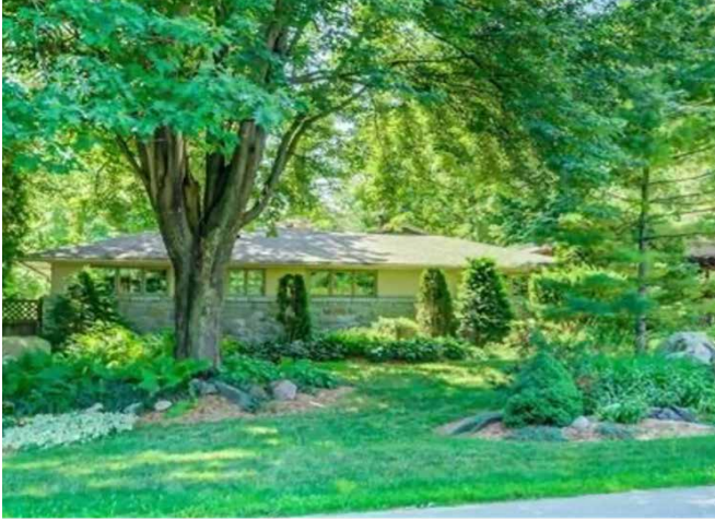
Figure 20: Ottawa home pre demolition
