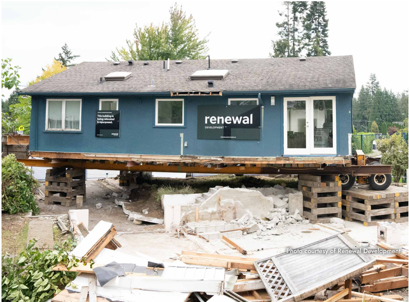
Figure 9: The Colwood Home being prepared for relocated to the Squamish Nation
